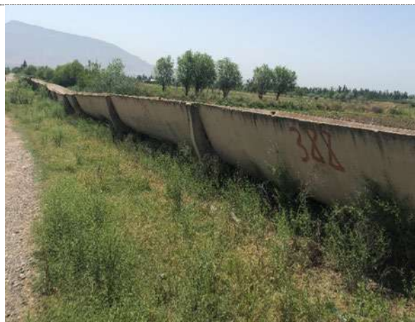
Secondary Pre-cast (tray) parabolic canal with failed sections is no longer used. About 4.51 km of PL4 will be rehabilitated under the project.
