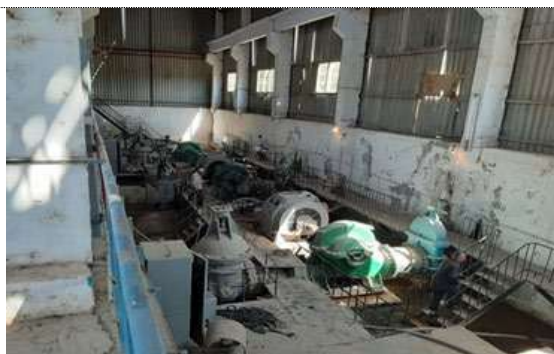
Pump Station Rasvet #6 at KM 649.8 of the Right Branch. It was constructed in 1972 and has 4 pumping units. It is 50% functional as 2 pumps not operable, as well as valves. The discharge 1,630 m long, 1,220 mm dia. steel pressure pipeline is badly deteriorated. This pumping station is one of two that will be rehabilitated and modernized under the project.
