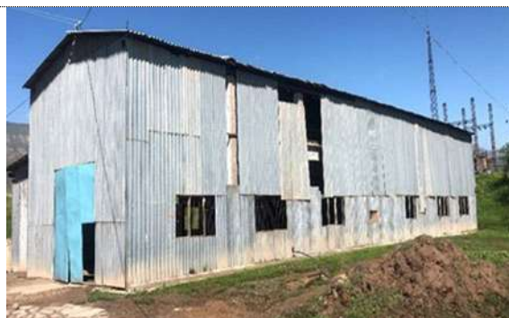
Pump Station Rasvet #6 at KM 649.8 of the Right Branch. It was constructed in 1972 and has 4 pumping units. It is 50% functional as 2 pumps not operable, as well as valves. The discharge 1,630 m long, 1,220 mm dia. steel pressure pipeline is badly deteriorated. This pumping station is one of two that will be rehabilitated and modernized under the project.
