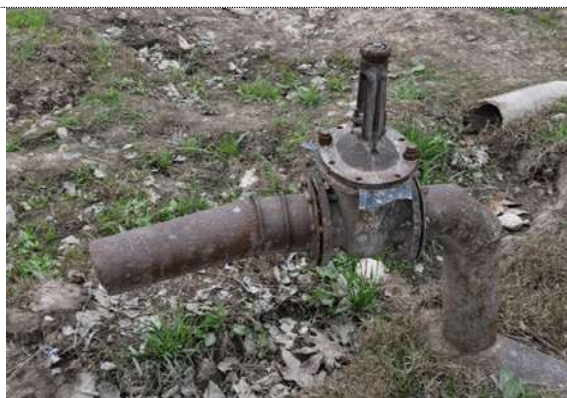
The old (1960s) steel hydrants for field crop irrigation will be replaced with modern hydrants that enable gated pipe and/ or hose irrigation.
