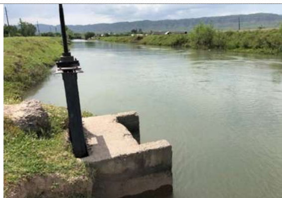
Gated Offtake #19 to a buried pipeline in WUA Chorgul command area. All the offtakes supplying the core area of 9,830 ha will be rehabilitated under the project.
