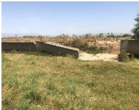
Secondary Pre-cast (tray) parabolic canal with failed sections is no longer used. About 4.51 km of PL4 will be rehabilitated under the project.
