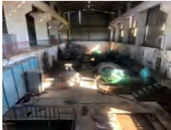
Photo 16 and Photo 17. PS Rassvet #6" Constructed in 1972. 4 pumping units. 50% functional as 2 pumps not operable, as well as valves; 1,630 m long, 1,220 mm diameter steel pressure pipeline deteriorated.
