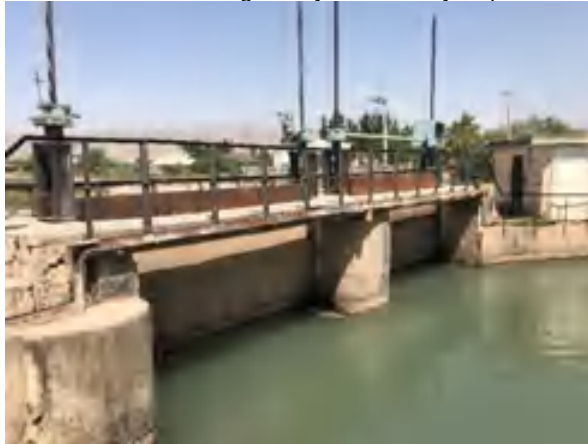
Photo 4. Check (cross regulator) Gates cannot be operated manually, and motors are broken. A truck crane is used. Gates and gate bearings need replacement.
