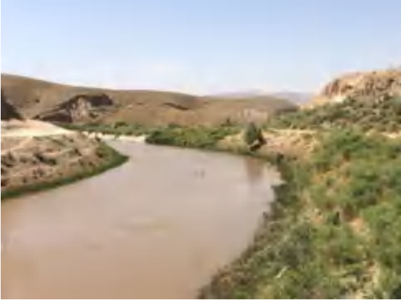
Photo 1. Right Branch Loikasai Bypass Channel – lining required.
