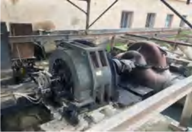
Photo 12 and Photo 13. PS #5. Constructed in 1968. 4 pumping units (1 small) 50% functional as 1 pump and 2 motors not operable; pressure pipeline deteriorated, electric cabling in poor condition.
