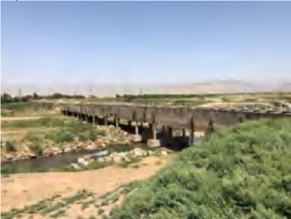
Photo 3. Aqueduct 140 m long and design capacity of 50 m 3 /s. Main problems are holes in troughs and scouring out of foundations for some of the supporting pillars.
