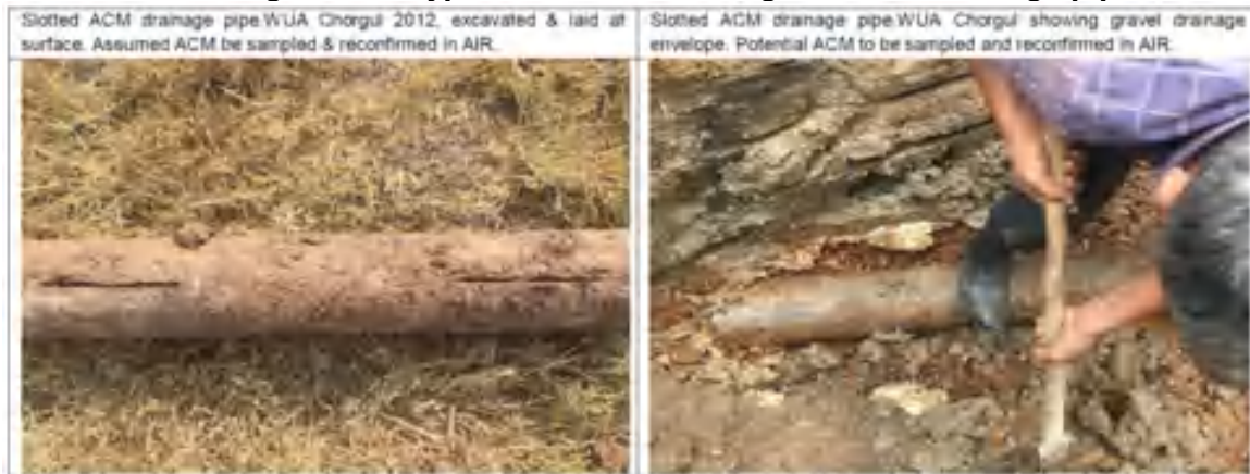
Figure 2-2. Typical condition of irrigation and drainage pipes.
