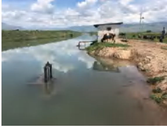
Photo 2. Outlet from Right Branch underwater as canal water level is raised high to try and convey required flow
