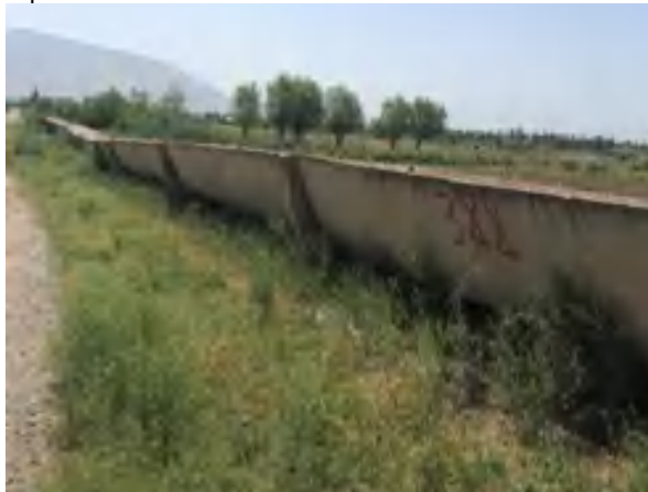
Photo 6. Flume or “Gravity” secondary canals leading from Right Branch comprise mostly pre-cast concrete flumes, some of which have now subsided and failed.
