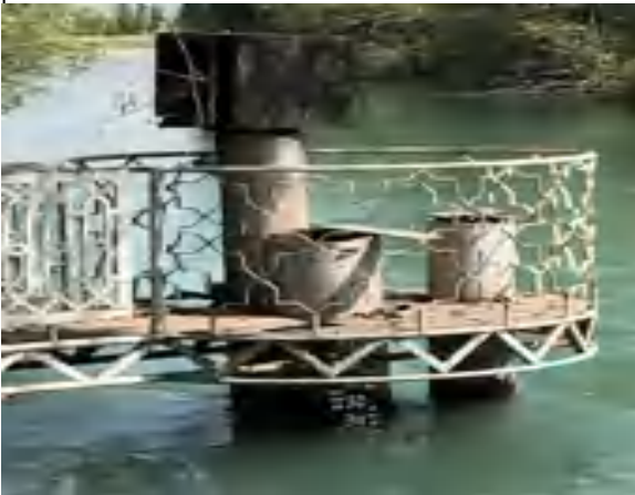
Photo 5. Gauging Station along Right Branch
