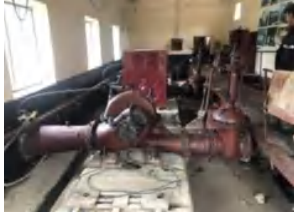
Photo 12 and Photo 13. PS #5. Constructed in 1968. 4 pumping units (1 small) 50% functional as 1 pump and 2 motors not operable; pressure pipeline deteriorated, electric cabling in poor condition.
