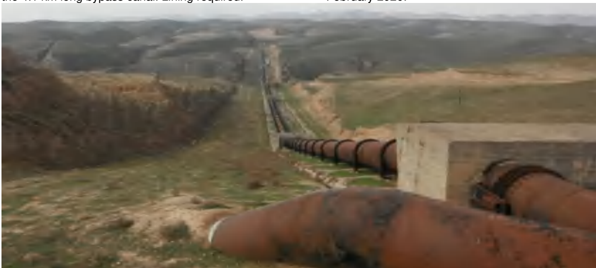
Photo 11. Shurchasoy Siphon 3 (1 No steel pipe and 1 new glass reinforced plastic (GRP) pipe). Either: (i) Construction of new bypass canal proposed, or (ii) a second siphon pipeline required. Capacity to be increased from 9-10 m 3 /s to 13-15 m 3 /s.
