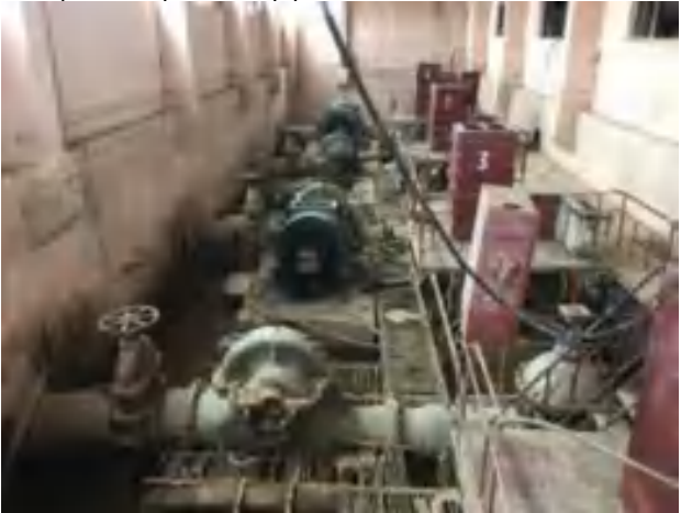
Photo 14 and Photo 15. PS #12. Constructed in 1976. 4 pumping units. 75% functional as 1 pump and 1 motor not operable, as well as valves; pressure pipeline deteriorated.
