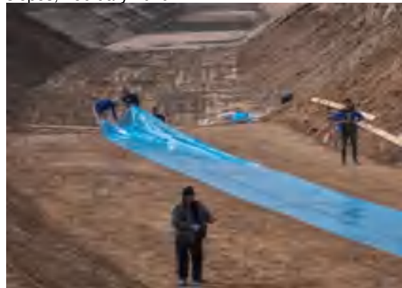
Photo 10. Short length of lining being constructed by ALRI in part of Loikasoi Siphon 2 bypass channel, February 2020.
