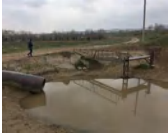
Photo 14 and Photo 15. PS #12. Constructed in 1976. 4 pumping units. 75% functional as 1 pump and 1 motor not operable, as well as valves; pressure pipeline deteriorated.
