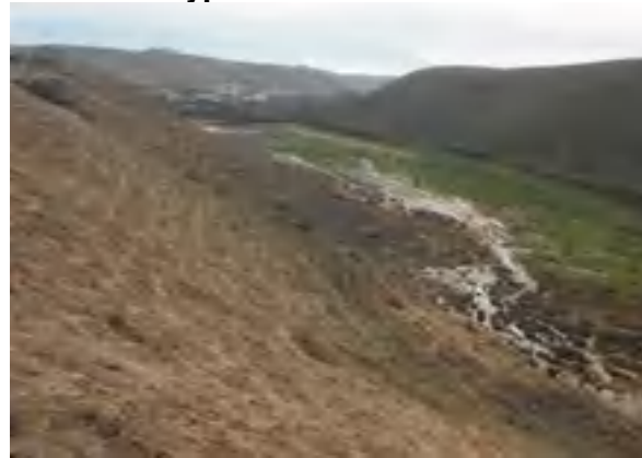
Photo 8. The bypass channels are unlined and seepage and small slip failures were observed in the downside slopes, February 2020.
